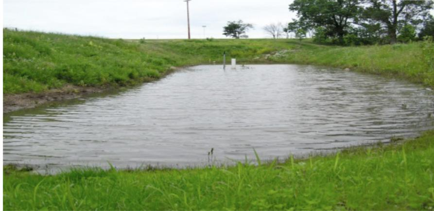
The dry detention ponds investigated drained, in most cases, far slower than the 48-hour drainage target for which they were designed. Sediment and under-drain design were the principal culprits of the drainage problems.
