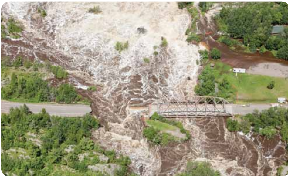
Severe flooding in June 2012 knocked out key infrastructure in northern Minnesota.
