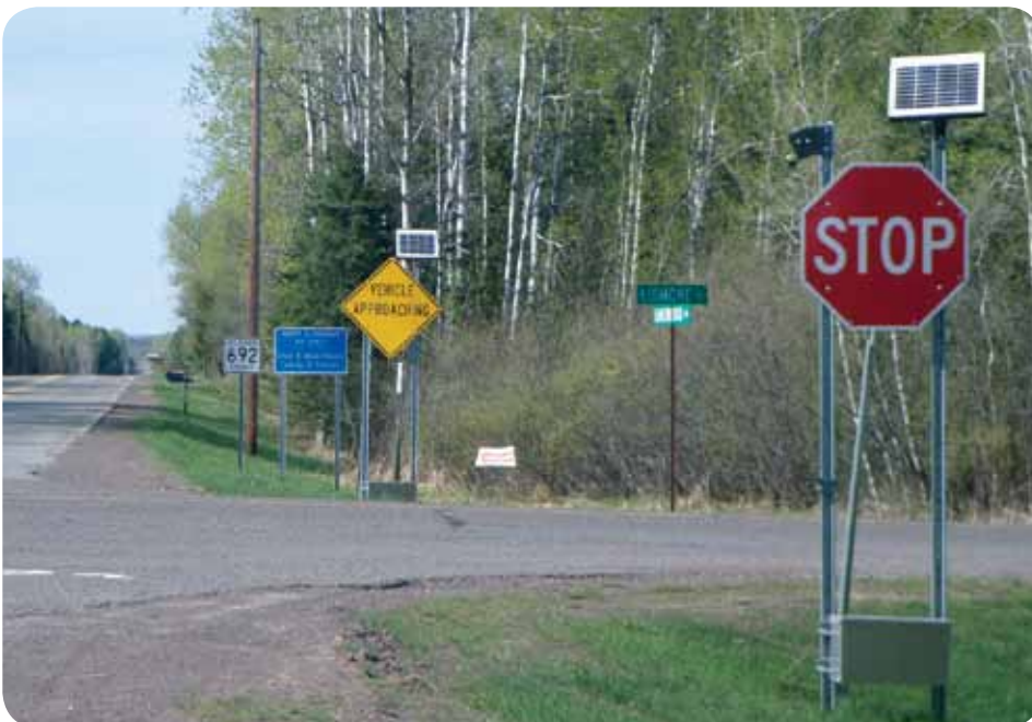
In the latest phase of the project, researchers removed the "When Flashing" label from the warning sign and added LED flashing lights to the existing stop sign.
