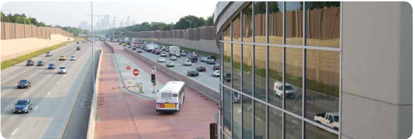
Buses leaving the 46th Street station in the median need to cross lanes to reach the next station located on the right side of the freeway.
