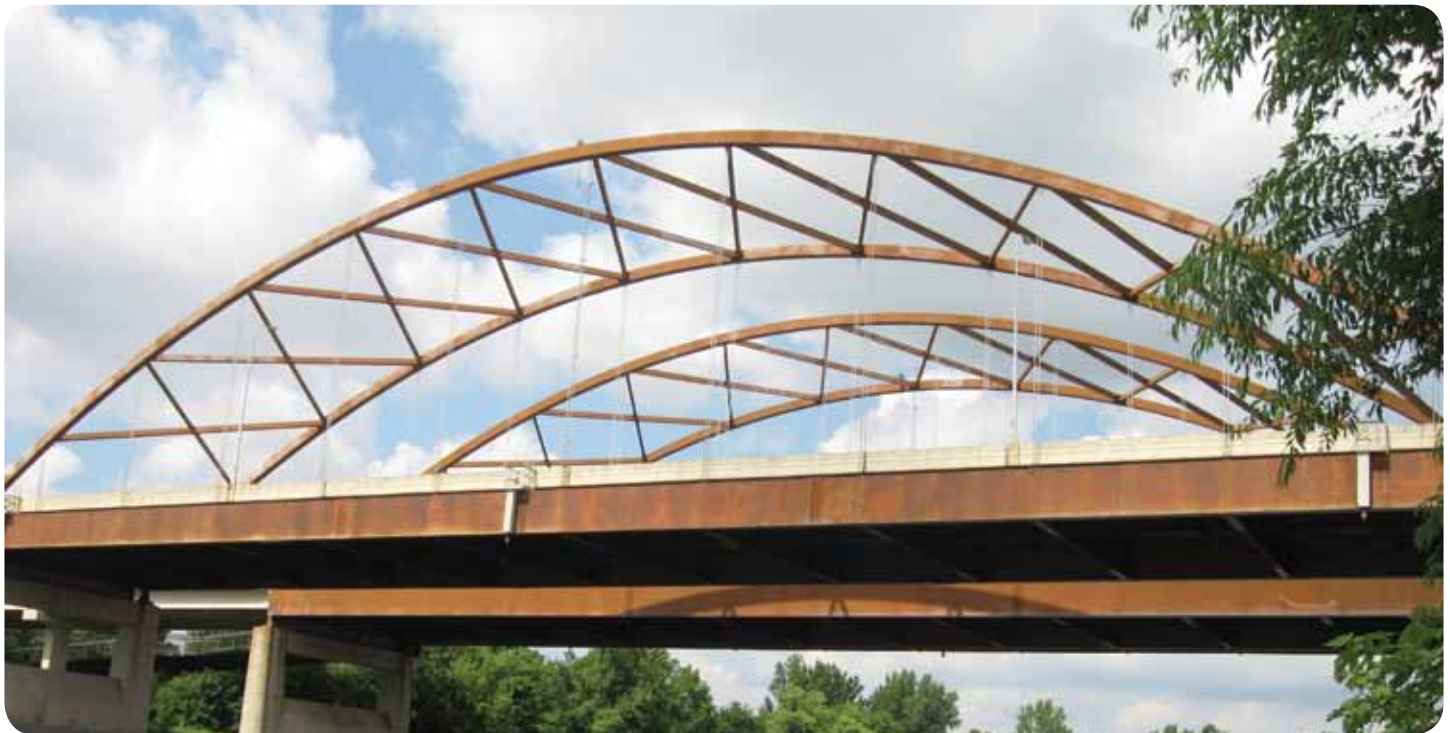
Acoustic sensors listen for potential problems—such as a bolt cracking—to monitor the health of a bridge.
